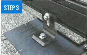
ATTACH L-FOOT TO RAIL
