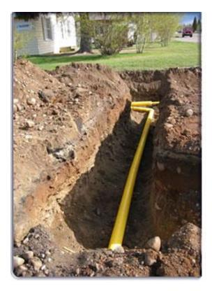
**6...** The gas is delivered to the distribution system thru 2 to 6 inch steel and medium density polyethylene pipes.
