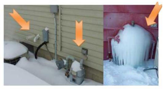
Accumulations of snow and ice from heavy snows, ice storms, snow and ice falling from rooftops, snow removal by shoveling and other equipment, faulty gutters, etc. may cause damage or failure to meters, regulators and piping due to stress conditions.
