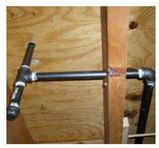
However, black iron pipe installation is time-consuming to install. Installers must cut the rigid pipe to specific dimensions and thread (manually or automatically) the pipe ends that will be connected together with appropriate black iron fittings sealed with approved pipe joint compound or Teflon tapes. Most black iron pipe projects are best performed by a professional installer or contractor.
